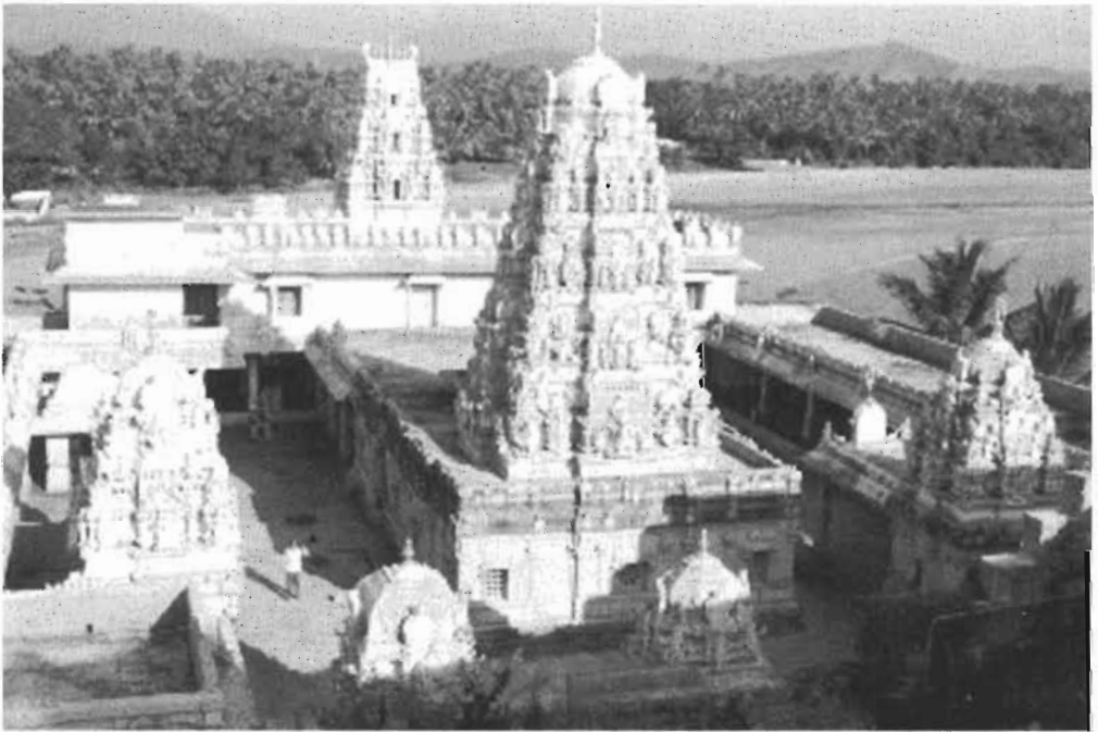
An aerial view of a Dravidian Style Temple, Murudeshwar
